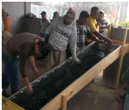
INSTALLING LATH
